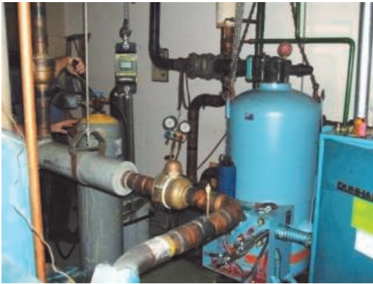
Pre and Post Pictures of Bitzer CSH8563-125-4PU Replaced Hartford Dunham Bush Vertical Screw Compressor 1215NHF6W4KBJ
