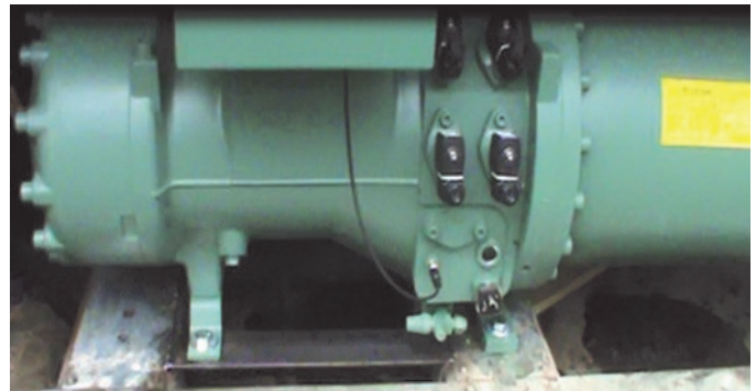
Re-used (2) existing mounting holes from McQuay and (2) New holes
