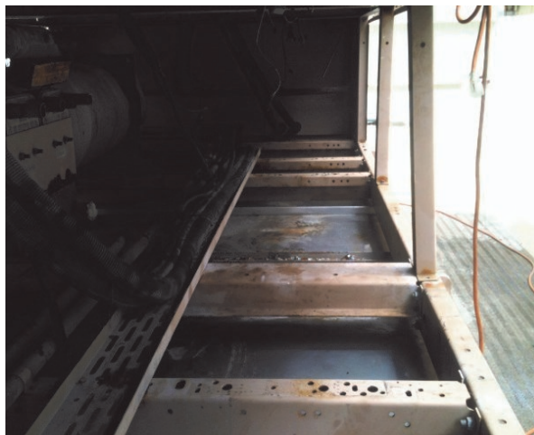
Base Frame cleaned and prepped for installation of BITZER CSH screws compressors
