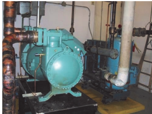
Pre and Post Pictures of Bitzer CSH8573-140-4PU Replaced Hartford Dunham Bush Vertical Screw Compressor 1215NHF6W4JBJOC
