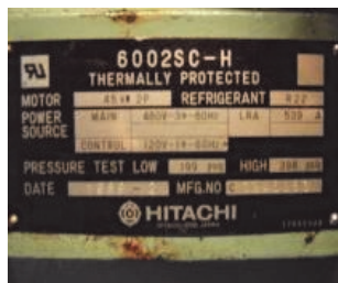
(4) 6002SC-H Screw Compressors (80 Horsepower)
