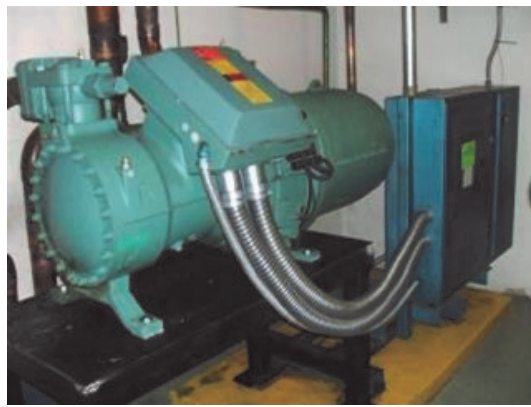
Pre and Post Pictures of Bitzer CSH8563-125-4PU Replaced Hartford Dunham Bush Vertical Screw Compressor 1215NHF6W4KBJ
