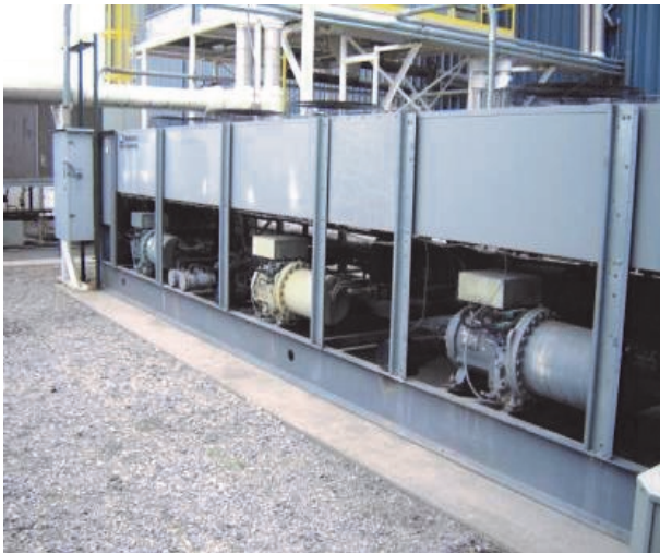
(4) 6002SC-H Screw Compressors (80 Horsepower)
