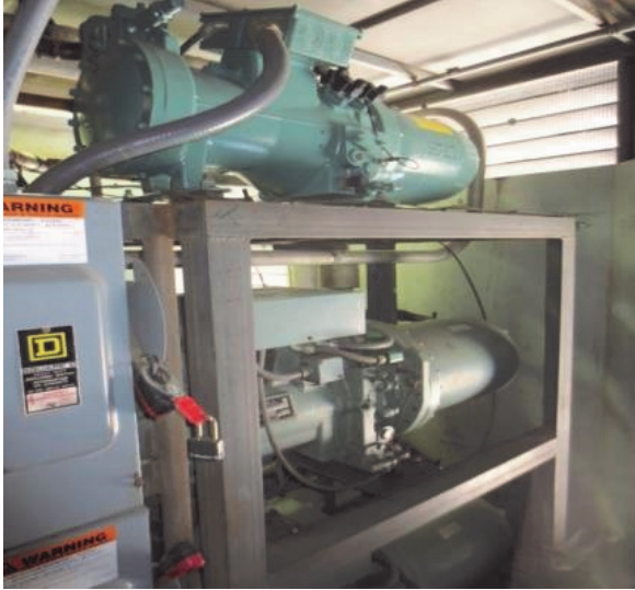
CSH6553-50-4PU CS Compressors (50 horsepower) CSH6563-60-4PU CS Compressors (60 horsepower)
