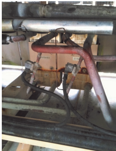
Economizer Heat Exchanger, Thermal Expansion and Solenoid Valve Removal
