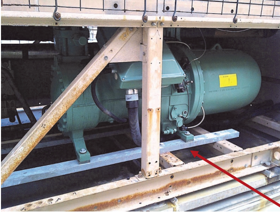
Added "U" Channel for Mounting of the CSH Bitzer Screw Compressor
