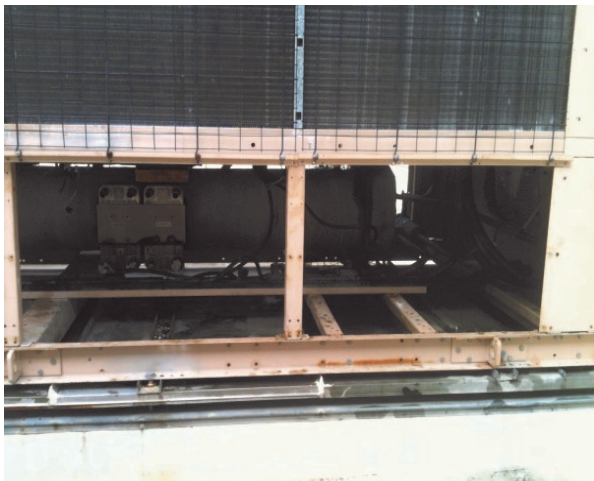
Base Frame cleaned and prepped for installation of BITZER CSH screws compressors
