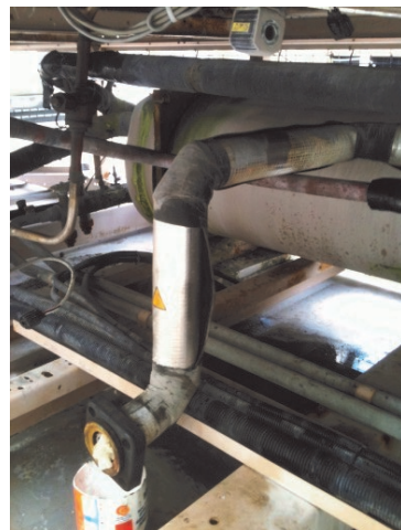
DXS45 compressors removed with existing suction and discharge piping shown
