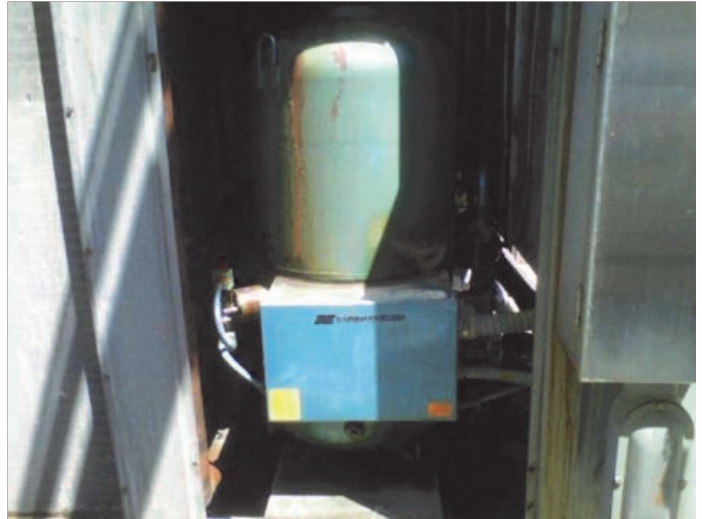
Pre and Post Pictures of Bitzer CSH8563-125-4PU Replaced Hartford Dunham Bush Vertical Screw Compressor 1215NHF6W4KBJ
