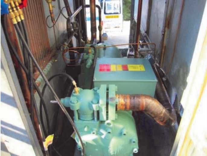
Pre and Post Pictures of Bitzer CSH8563-125-4PU Replaced Hartford Dunham Bush Vertical Screw Compressor 1215NHF6W4KBJ
