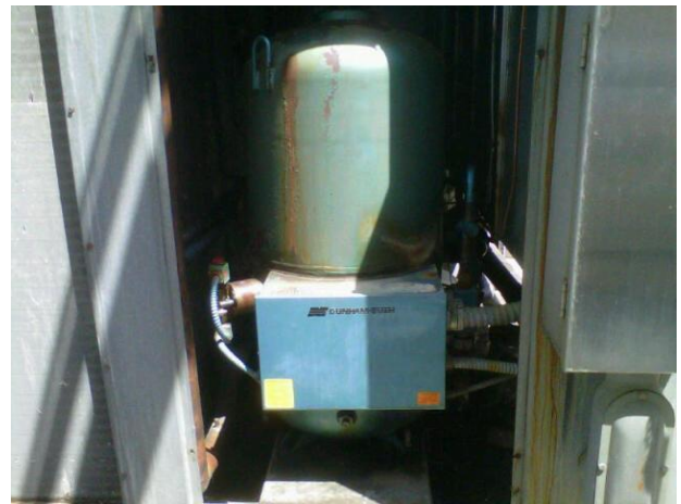
Post and Pre Pictures of Bitzer CSH7573-90-4PU Replaced Hartford Dunham Bush Vertical Screw Compressor 1117NHF6X6K
