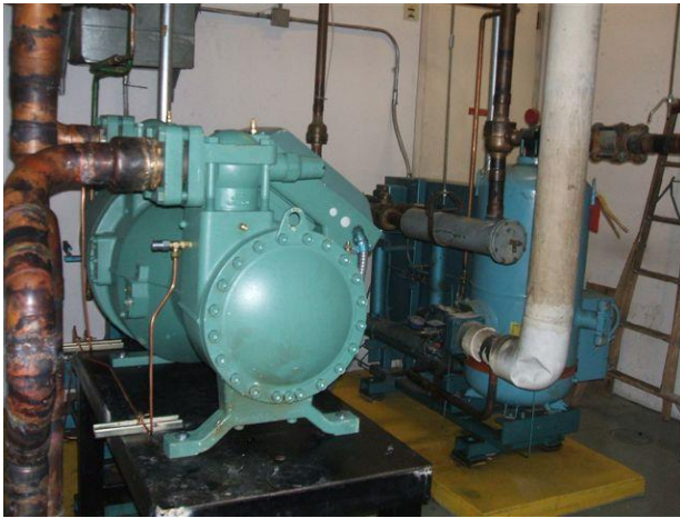
Post and Pre Pictures of Bitzer CSH7573-90-4PU Replaced Hartford Dunham Bush Vertical Screw Compressor 1117NHF6X6K
