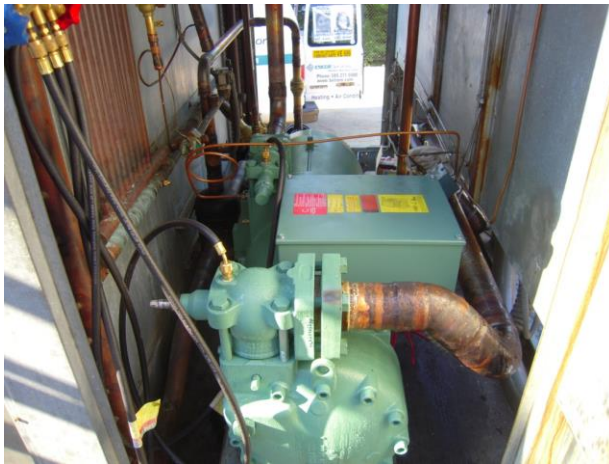
Post and Pre Pictures of Bitzer CSH7573-90-4PU Replaced Hartford Dunham Bush Vertical Screw Compressor 1117NHF6X6K
