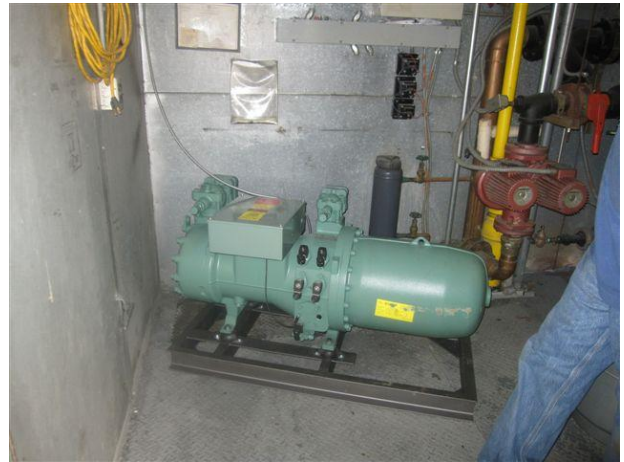
Post and Pre Pictures of Bitzer CSH7573-90-4PU Replaced Hartford Dunham Bush Vertical Screw Compressor 1117NHF6X6K
